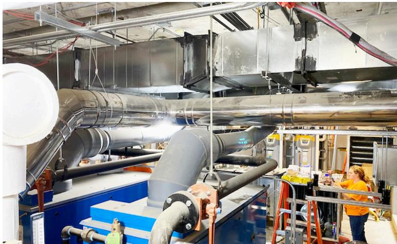
While Klein said that maneuvering very wide diameters of the double-wall duct was challenging due to the tight space, the installation team found the 24-in and under prefabricated duct easier to install than welded black iron. "Once you get the hang of it the install goes well!"
