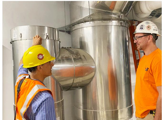
Chris Klein, Project Manager for Smith & Oby, explained “Logistically it just made sense to use one type of duct.” He also used DuraVent pre-fabricated flue duct for venting three Patterson-Kelley condensing hot water boilers on the project. DuraVent's product lines of specialty duct are UL listed for boiler, engine exhaust and grease duct applications which allowed for one source of product and design support.
