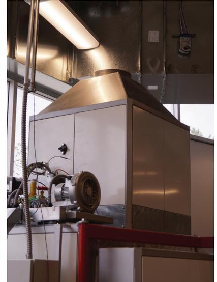
Robin instructed fabricators at Northwest Sheet Metal's shop in Surrey, British Columbia, to make stainless steel sleeves to fit around the single wall vent. Workers were able to install, as approved by Security Chimney engineers, the 2-piece half-circle sleeve sections and insulation around the single wall sections after all the exhaust vent was installed. In addition, Security Chimney custom fabricated several anchor plates to accommodate the existing structural steel supports.
