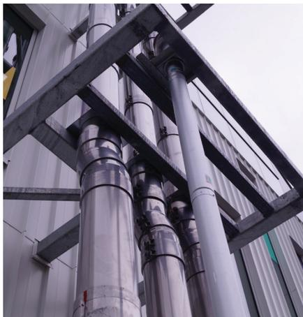
Robin was impressed with Secure Stack Pros unique self-centering design and coupling configuration that requires only one locking band and a standard, high-temperature silicon sealant for secure connection.
