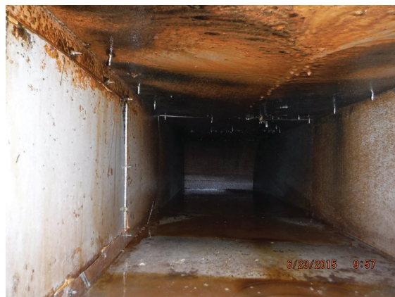
Square kitchen exhaust duct that has been screwed together in lieu of welding, opening the door for leaks through seams and screw holes. Photo courtesy of Derby Pressure Wash, Louisville, KY
