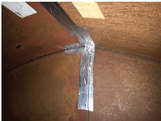
Grease duct seams inappropriately covered with duct tape (typically used for residential clothes dryer exhaust duct), presumably applied to pass a leak test. Photo courtesy of Derby Pressure Wash, Louisville, KY
