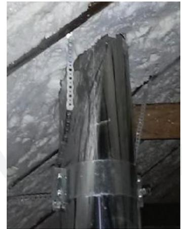
This example shows spray-foam insulation in direct contact with the chimney, which is a serious potential fire hazard!
